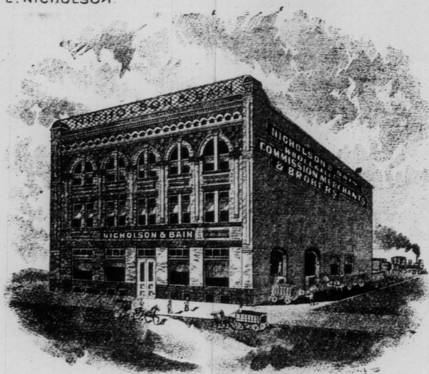
BANNATYNE ST. EAST TRANSFER TRACK.
