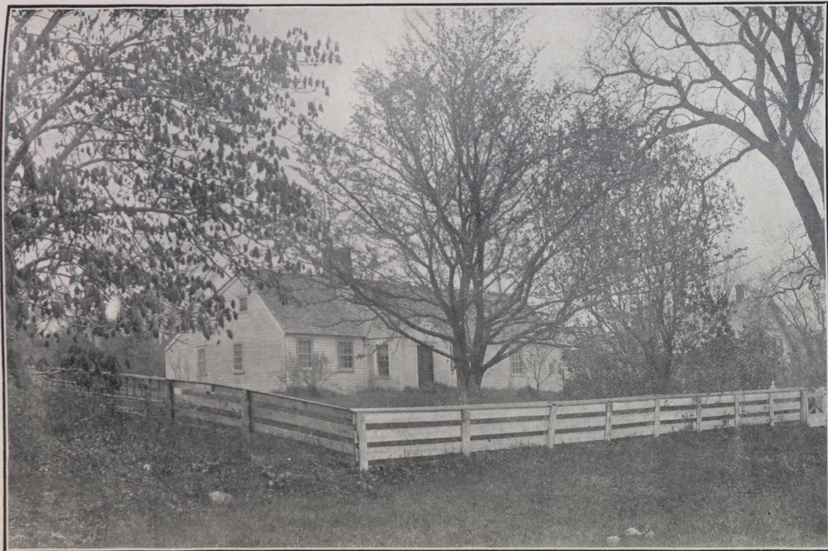
THE HOME OF JEREMIAH POTE, BROUGHT TO ST. ANDREWS, AND ERECTED ABOUT 1784,
