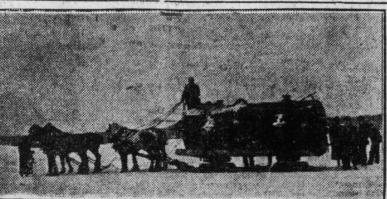
Carting machinery into the Porcupine. Boiler for the West Dome crossing Frederickhouse Lake. Freight will be hauled over the corduroyed roads right until the break-up.
