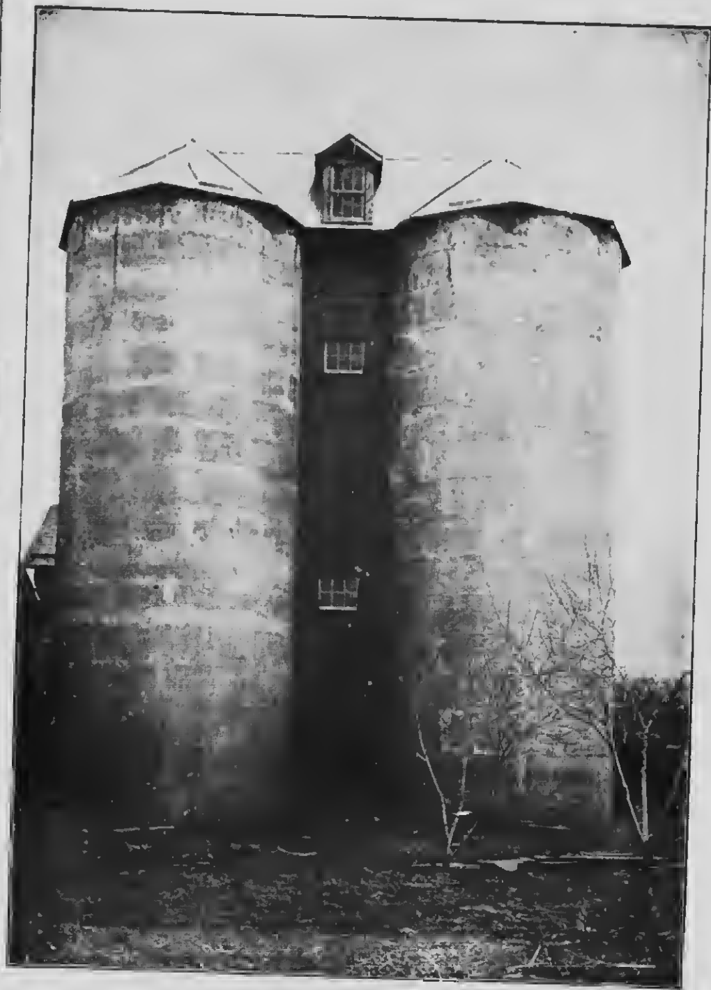
Showing two Concrete Silos with a Chute between them.
