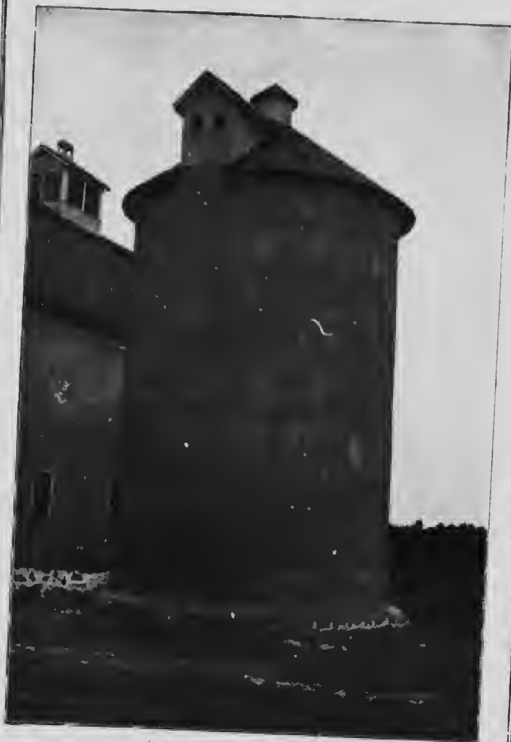
A Silo Built of Cement Blocks.
