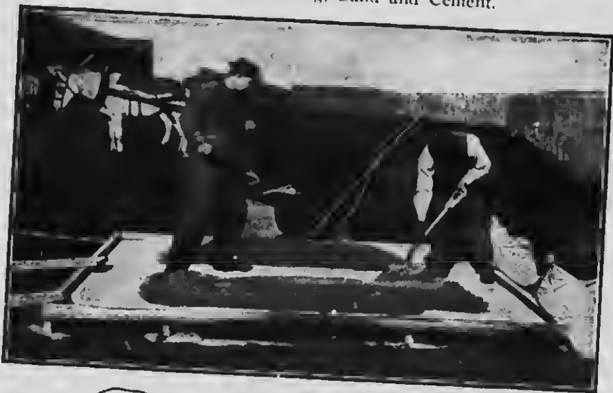
Fig. 6.—First Turning, Sand and Cement.
