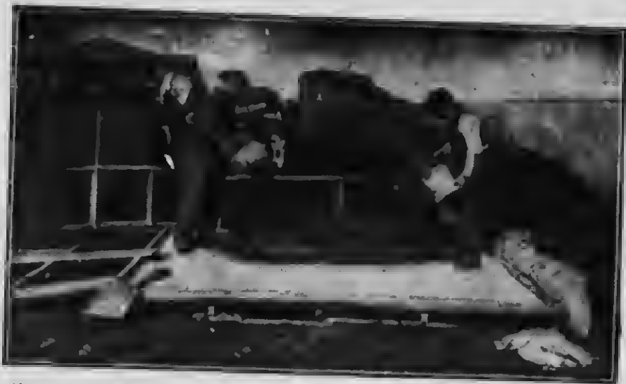
Fig. 10.—Placing the Water on the Stone (or Gravel) which is on Top of the Mixed Sand and Cement.
