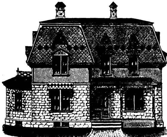
Fig. 1.—FRONT VIEW OF HOUSE.
