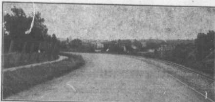
This is Merriton Road in St. Catharines, an important thoroughfare running through the manufacturing district between St. Catharines and Merriton, resurfaced with 'Tarvia'. Road width, 'Tarvia' is not cut to 10:1.
