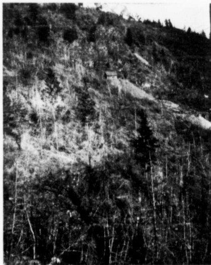
BEN D'OR MINE—SHOWING TUNNELS.
