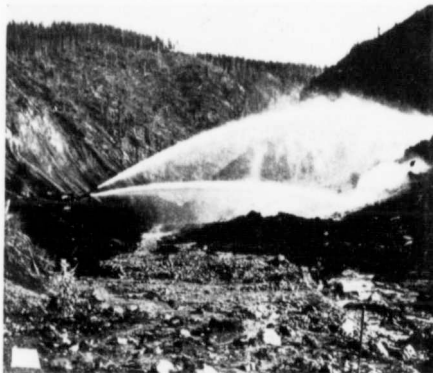
Two 8-inch streams opening up Pit No. 2, at S. Fork Mine, Cariboo.
