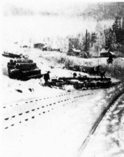
OFFICE AND BOILER BUILDINGS AT SNOWSHOE MINE.
