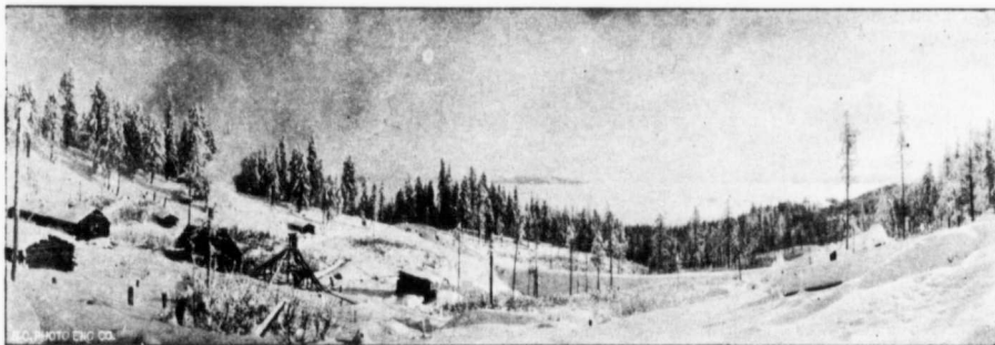
SNOWSHOE MINE ABOVE THE CLOUDS, VALLEY OF KETTLE RIVER IN BACK GROUND.
