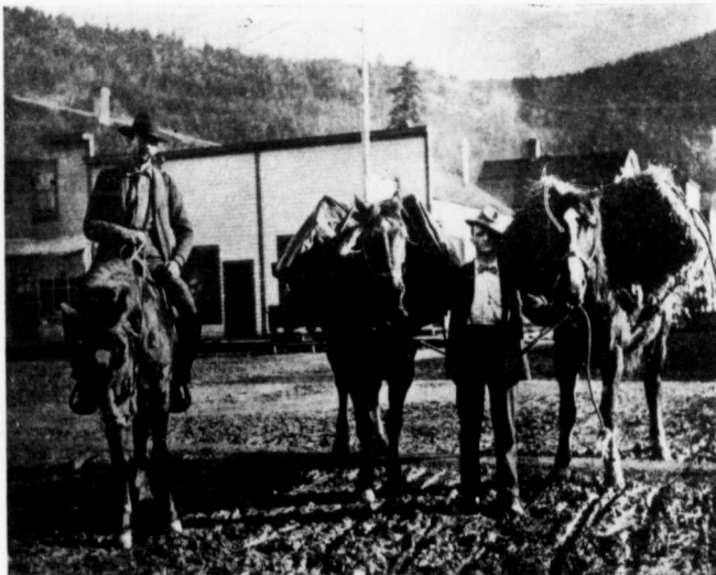
METHOD EMPLOYED OF TRANSPORTING SUPPLIES TO THE SLOCAN LAKE MINE.
