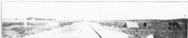
End of Steel, Preeceville, Sask.
