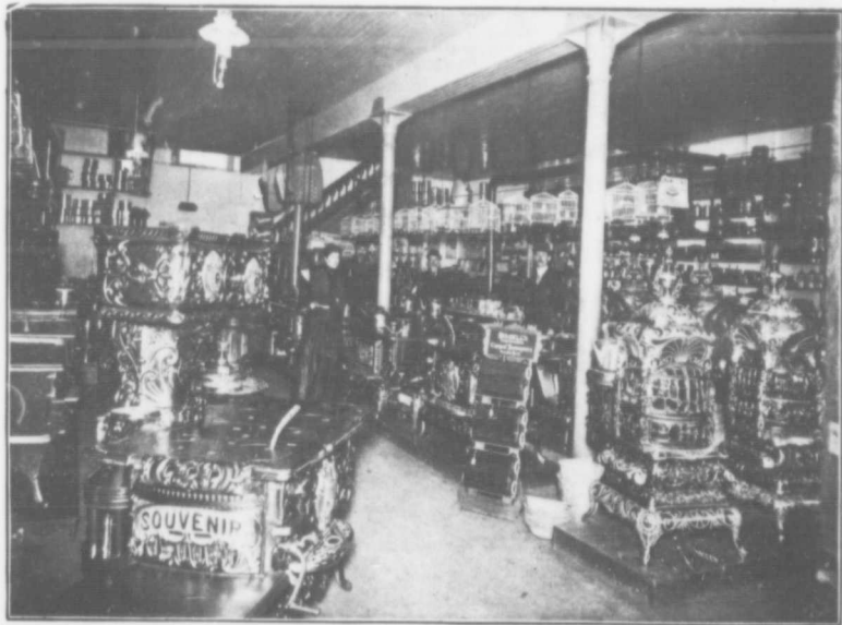
Interior View of Wm. Wyatt & Son's Stove and Housefurnishing Store, Nos. 385-387 Talbot Street, London.
