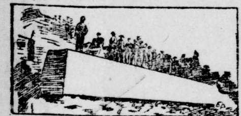
BLOCK OF GRANITE FOR ONE OF THE COLUMNS—WEIGHT 310 TONS; LENGTH, 67 FEET; HEIGHT, 84 FEET; WIDTH, 7 FEET.
