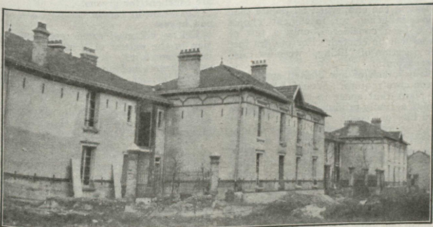
PHOTO SHOWS some of the workingmen's homes erected in the rebuilt city of Reims, France. Reims has a socialistic town council, which has just approved the expenditure of several hundred million francs for reconstruction according to plans of architects in charge of the work.
