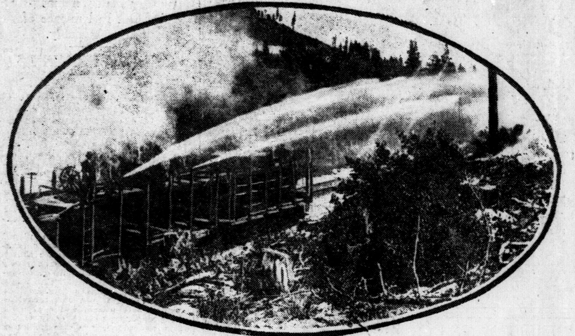
Trains are now being equipped with fire fighting apparatus and sufficient water capacity to battle a stubborn blaze for a full hour.
