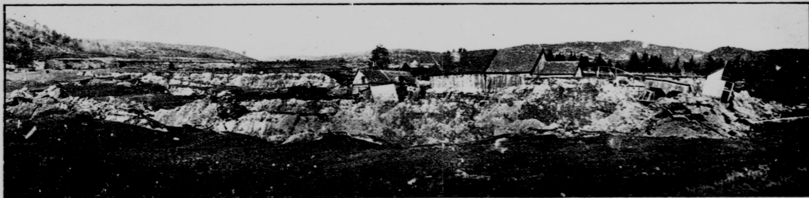
View looking west, — showing Clément's house and outbuildings and the uneven surface of the disturbed area.
