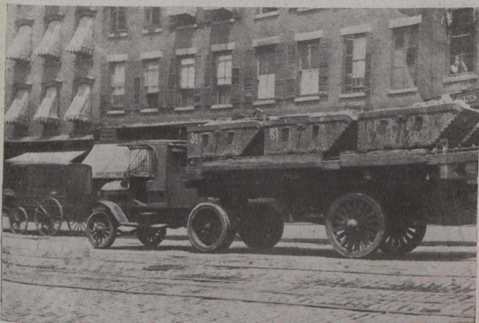
Type of Heavy Trailer Carrying 15 to 18 Tons of Broken Rock Which Caused Excessive Damage to Pavements.
