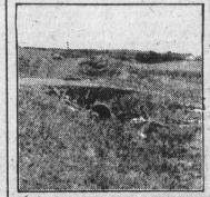
Method of Carrying Terrace Water Under a Roadway by Means of a Culvert.
