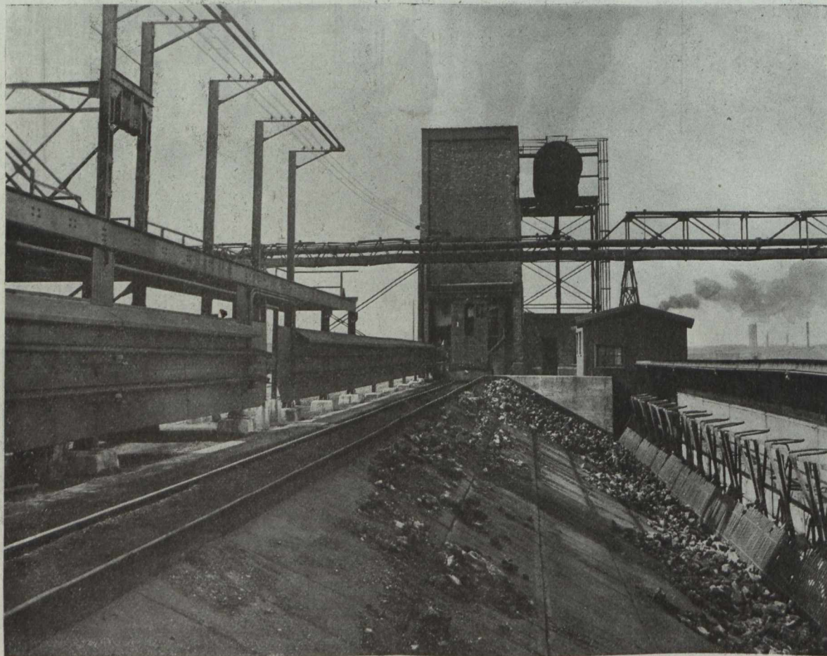
Fig. 4—Quenching a charge of coke. Coke-wharf on the right.
