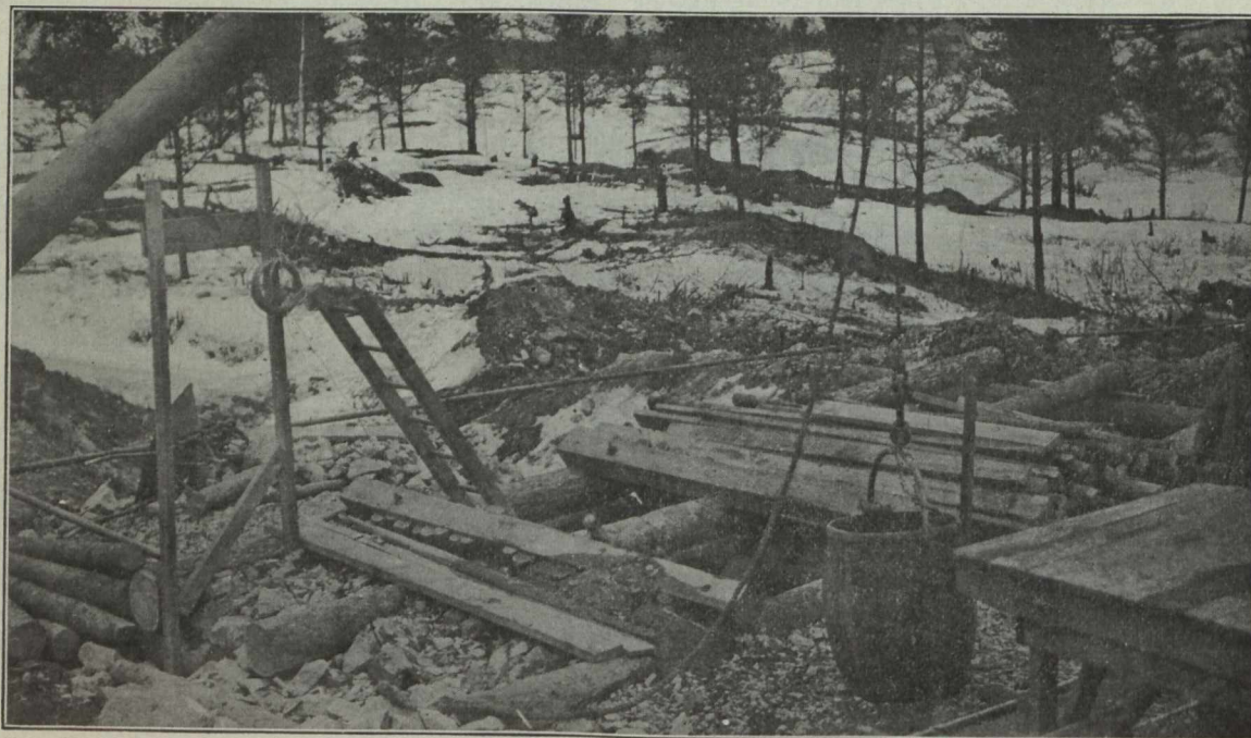
Shaft on No. 3 Vein, Tough-Oakes Mine, Kirkland Lake
