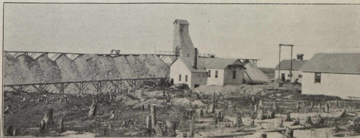
Shaft House and Stock Pile, Acme Mine
