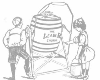
Bicycle Ball-bearings and rigid stand make the "LEADER" easy running—and there is nothing to interfere with pail being placed beneath bar to drain off the butter-milk.
