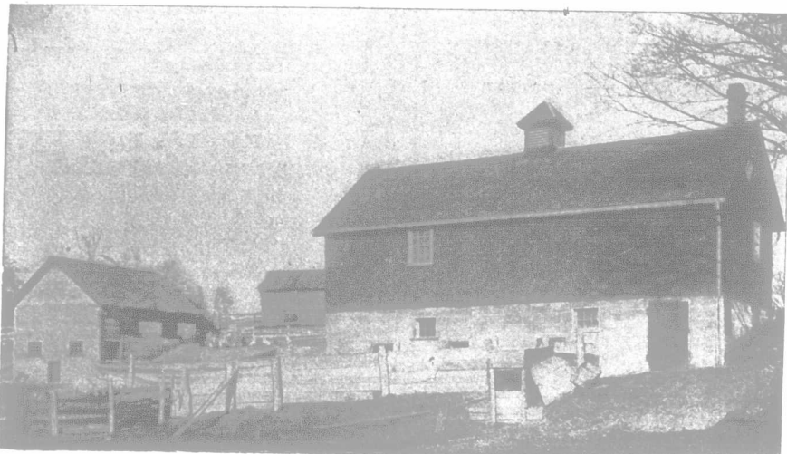
THE HENHOUSE. Wall, from foundation to peak, built with THOROLD CEMENT.
