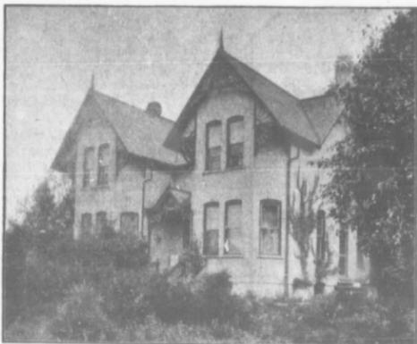
Farm Home of Mr. Clement White, Lambton Co., Ont., 26x36 ft. outside measurement—Kitchen 10x18 ft., 9 ft. ceilings. Built with hollow brick wall on stone foundation.
