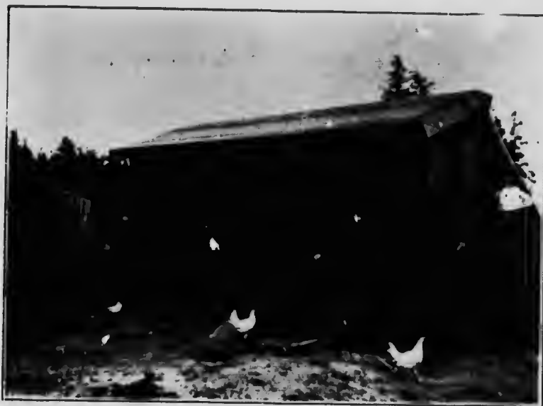
Fig. (13.) Small house, suited to Coast conditions. The kerosene can was inserted in the wire screen to allow birds egress and ingress, and as a protection against vermin.
