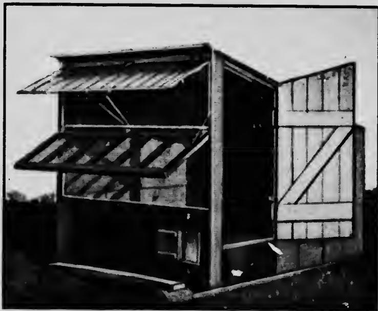
Fig. (18.) A good type of colony house. Measurements, 6 feet long, 8 feet deep, 6 feet 6 inches in front, 2 feet 6 inches rear. Colony houses can be hauled to any part of the ranch, thus giving young or old stock opportunity to range on clean soil. Can be used as cockerel, pullet, or breeding houses after chickens are matured. The top shutter or board window makes a splendid hood or rain-shield and can be changed to a muslin-curtain screen if desired.
