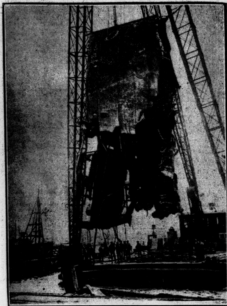
Iron is short in Germany, and they are salvaging old ships to get the metal. This picture shows a derrick pulling up the hull of a ship sunk ten years ago in the Kiel Canal.
