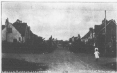
Inexpensive Roadway on Residential Street
