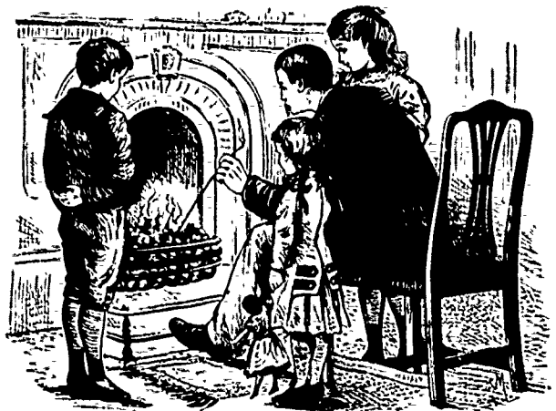
A VERY SMALL GAS-FACTORY.
