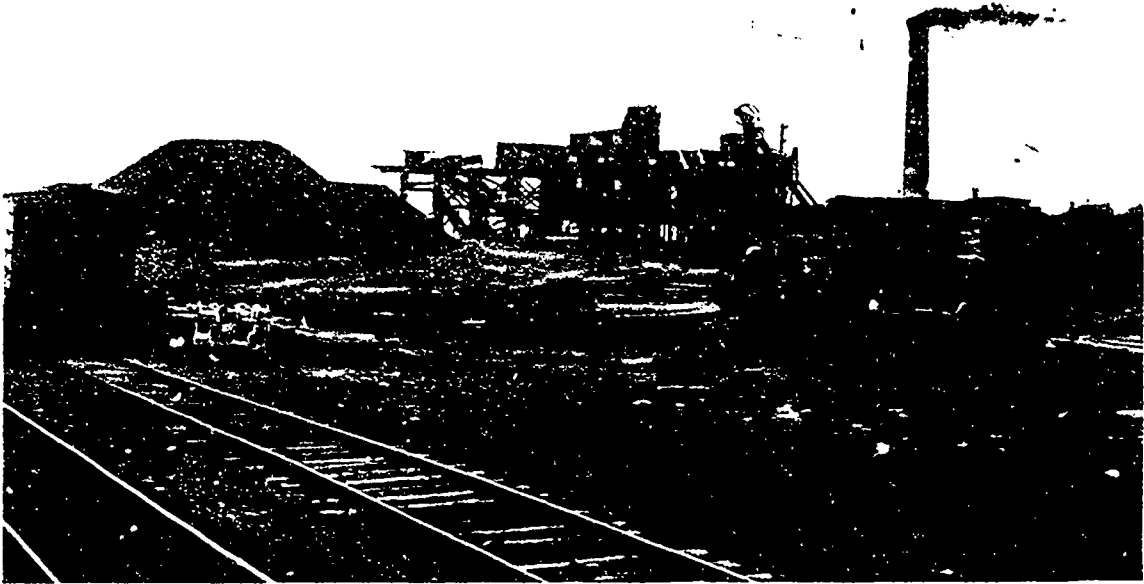
BANK-HEAD INTERNATIONAL COLLIERY OF THE DOMINION COAL CO.
