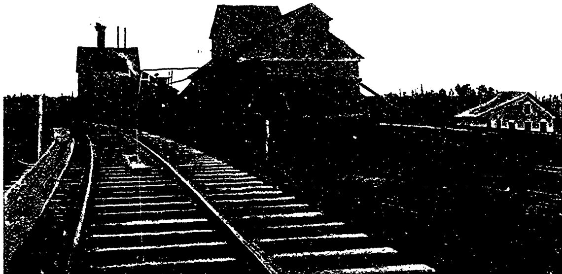
COAL WASHING PLANT ON THE MAIN LINE OF THE SYDNEY & LOUISBURG RY., SEVEN MILES FROM GLACE BAY, C.B.
