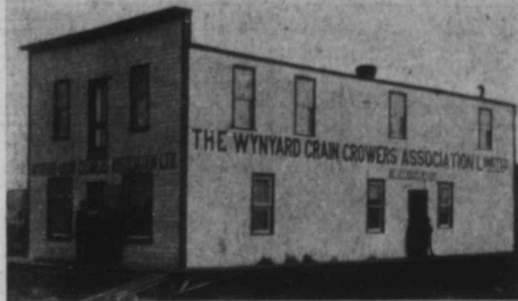
The Offices of the Wynyard G.G.A. include a Rest Room for the Women. The rest room and club room of the W.S.G.G.A. is also in this building. The entrance is by the side door. This is a splendid example of the co-operation between our farm men and farm women.
