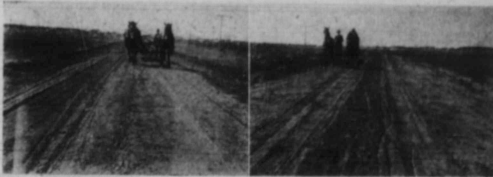
THE GRAVEL ROAD DRAG IN ACTION
