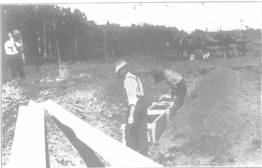
Putting in a Plank Culvert on Eighteen Foot Roadway
