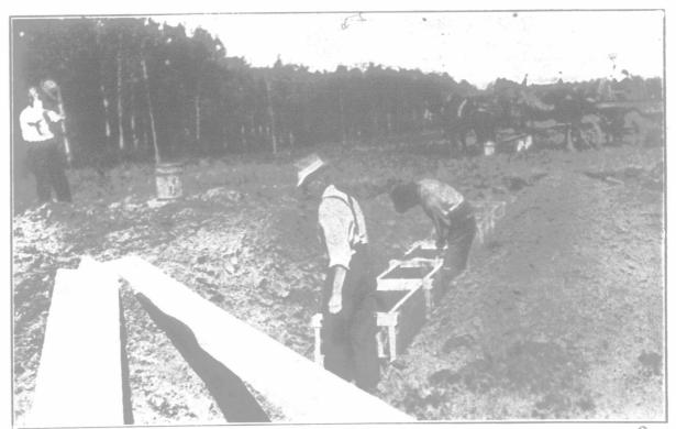
Putting in a Plank Culvert on Eighteen Foot Roadway In many districts cement tile or some material other than wood is being used
