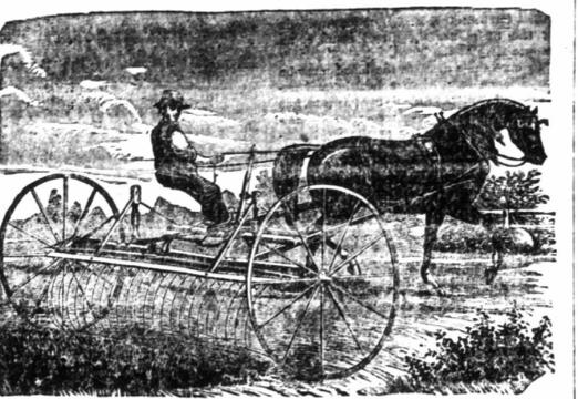
The WHEELS are of the STRONGEST POSSIBLE MAKE consistent with moderate weight. They have White Oak and Hickory Spokes, best Iron and Iron Hubs.
