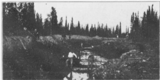
FINISHING THE DITCH.
