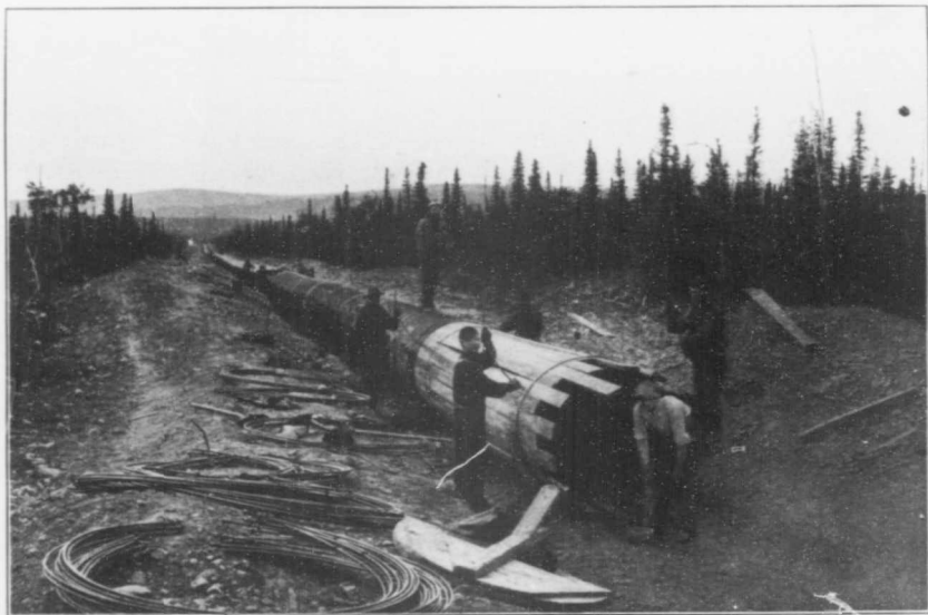
ASSEMBLING STAVE-PIPE ON THE LINE OF THE YUKON DITCH.
