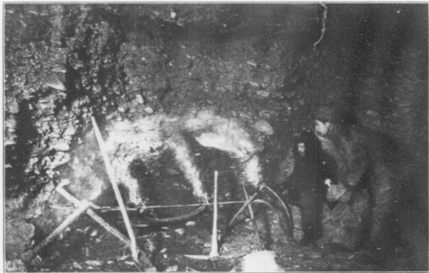
STEAM-POINTS IN PLACE UNDERGROUND.
