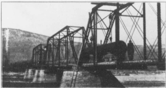
PIPE CROSSING THE KLONDIKE.
