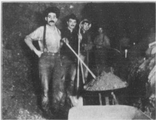
IN A DRIFT MINE.
