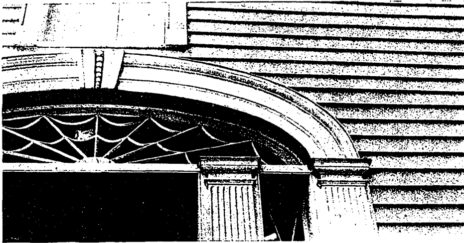
DOORHEAD: OLD COLONIAL HOUSE, GEORGEVILLE, QUEBEC.
