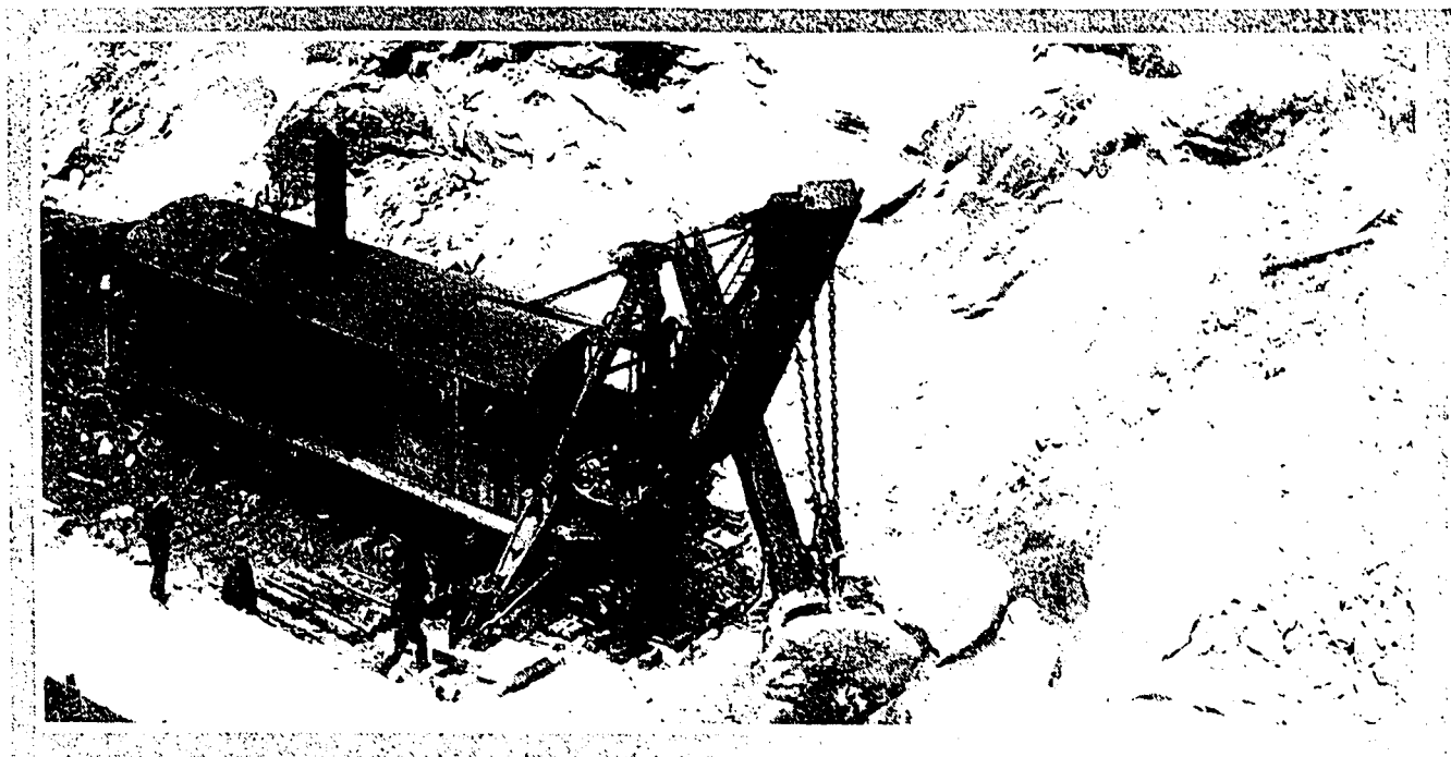
RAILWAY CONSTRUCTION WORK, VANCOUVER
