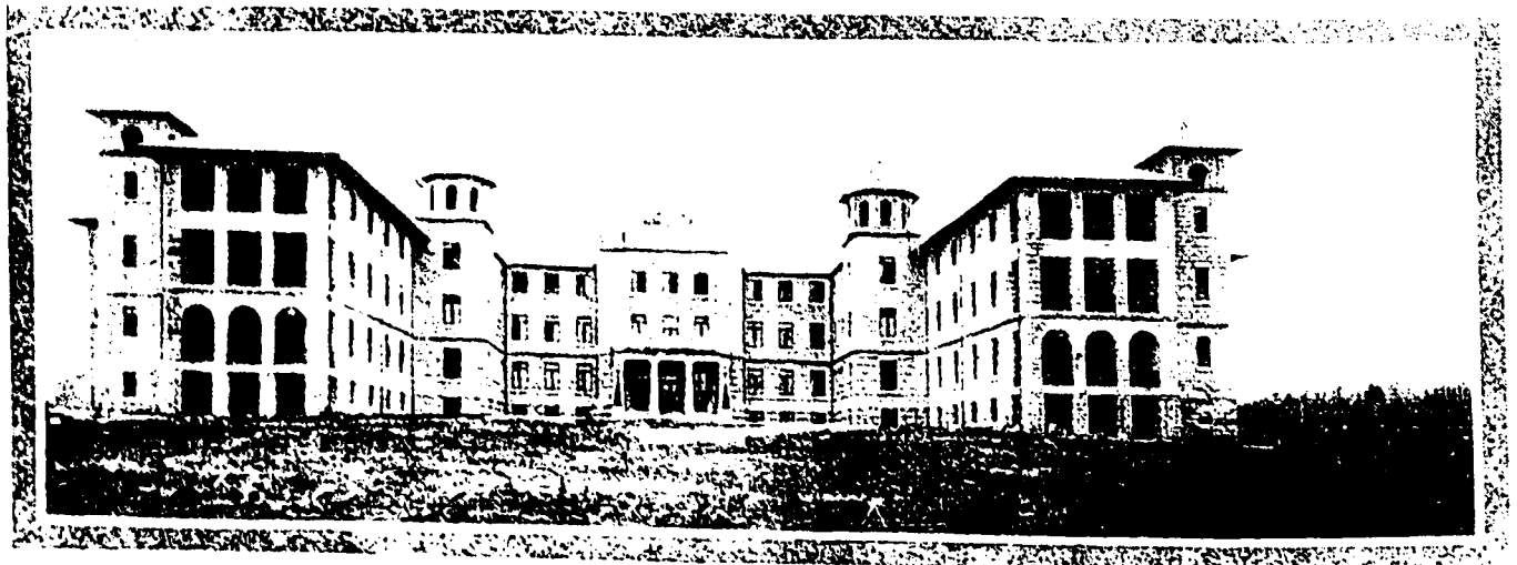
GENERAL HOSPITAL, VANCOUVER
