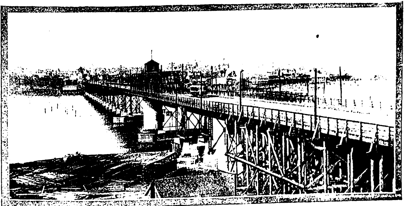
GRANVILLE STREET BRIDGE OVER FALSE CREEK, VANCOUVER
