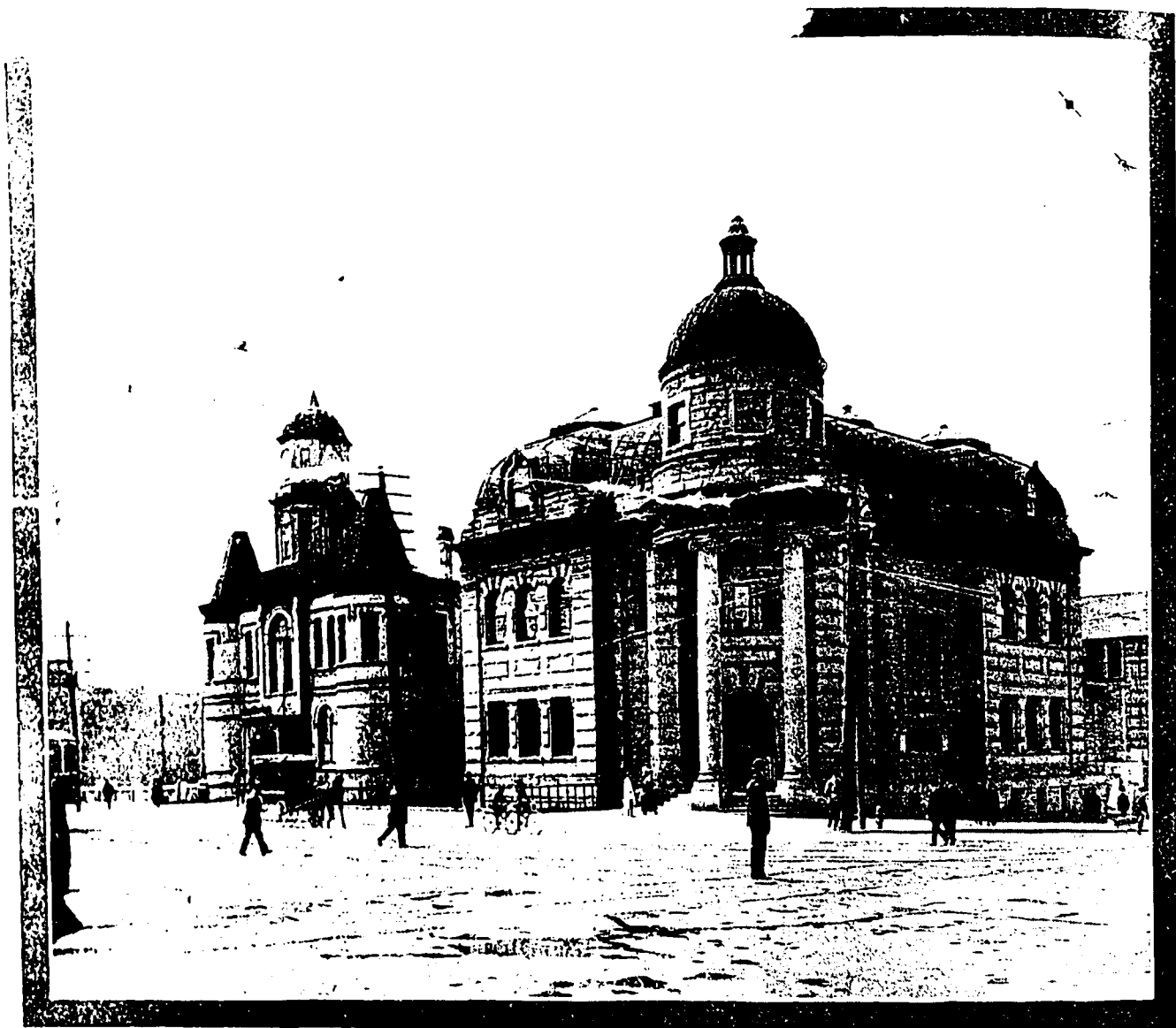
CITY HALL (SOON TO BE REPLACED BY A NEW BUILDING) AND CARNEGIE LIBRARY, VANCOUVER
