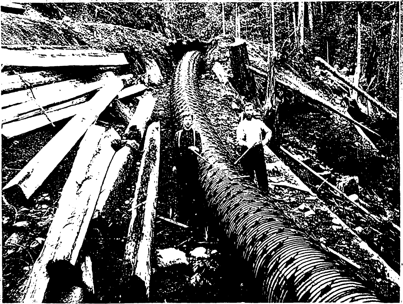
BIG WOODEN PIPELINE LEADING DOWN FROM THE SEYMOUR INTAKE THIS MAIN IS THIRTY-SIX INCHES IN INSIDE DIAMETER
