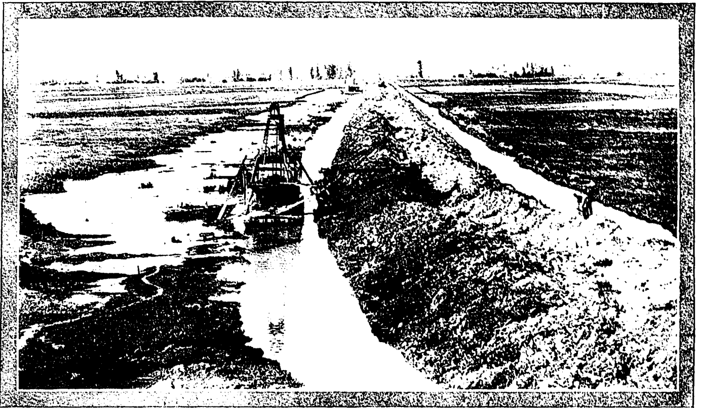
THE MAKING OF THE GRADE, NEAR VANCOUVER
