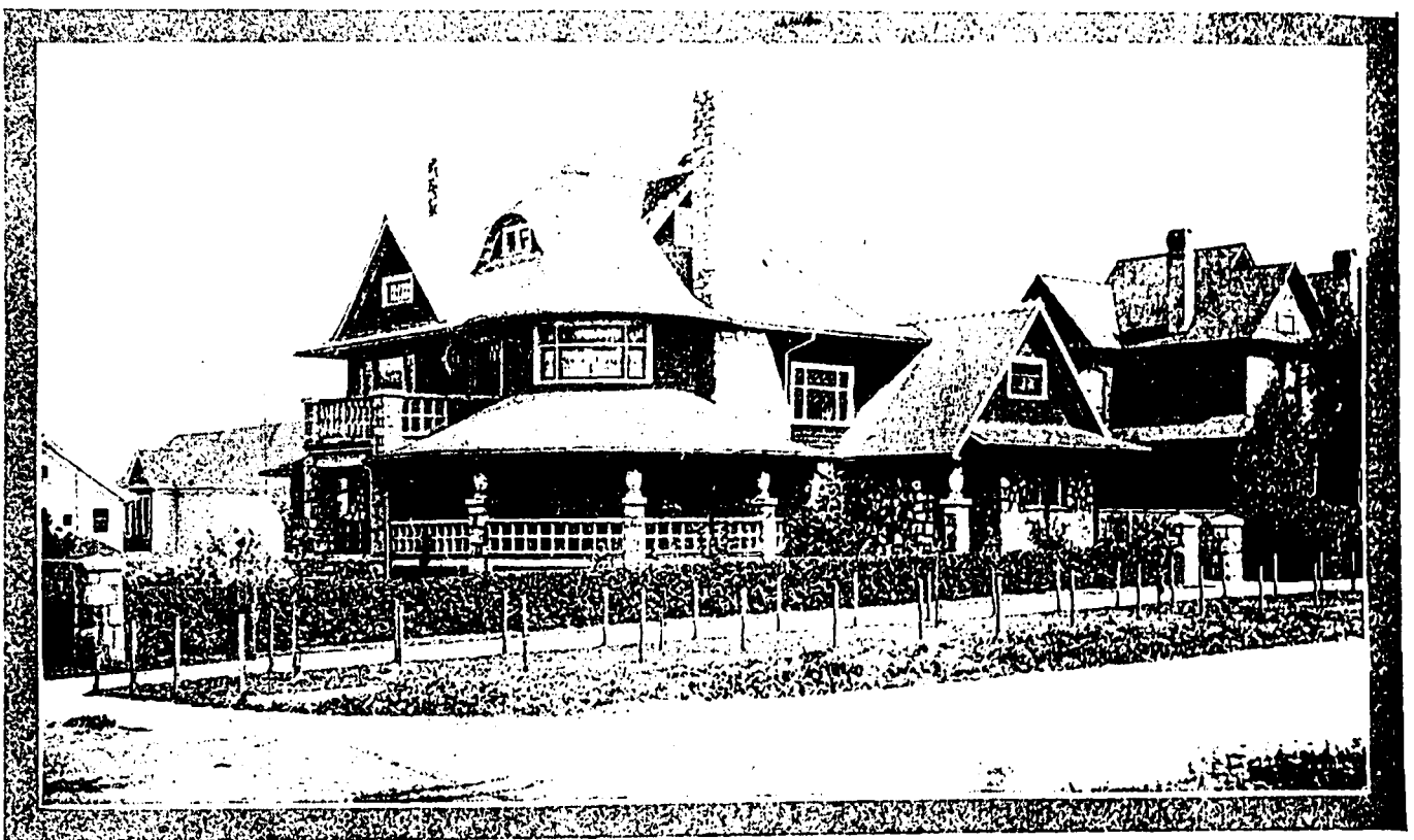
RESIDENCE, WEST END, VANCOUVER
