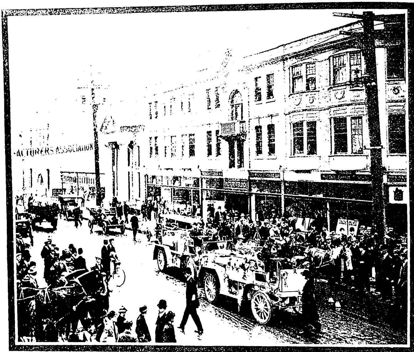
SOME OF THE MOTOR EQUIPMENT, VANCOUVER FIRE BRIGADE
