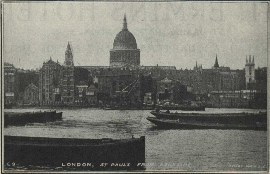
ST. PAUL'S, AS SEEN FROM THE SOUTH SIDE OF THE RIVER
