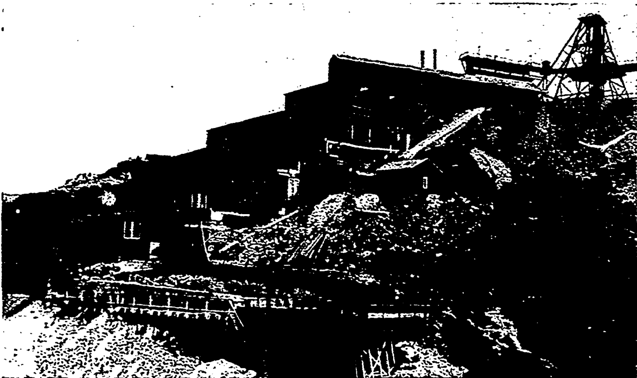
Concentrating Mill, Morenci, Arizona—Power furnished by three 50 H P. Gas Engines.
