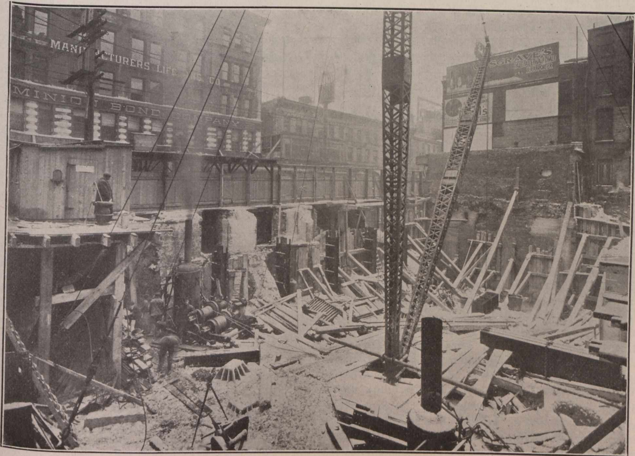
Fig. 1.—Showing Stage of Work on January 15th, 1914.
