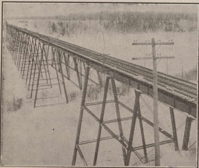
Fig. 1.—Viaduct Before Reinforcement.
