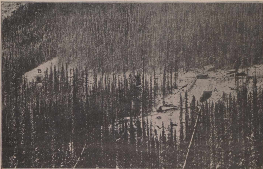
Fig. 5. Upper and lower portals spiral tunnel No. 2.
