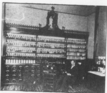
Dispensary, St. Joseph's Hospital, Peterborough.
