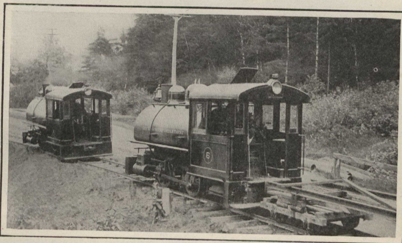
Building Toronto's first civic street car lines. These miniature engines are used to haul work trains with excavated material where the grading is being done.
