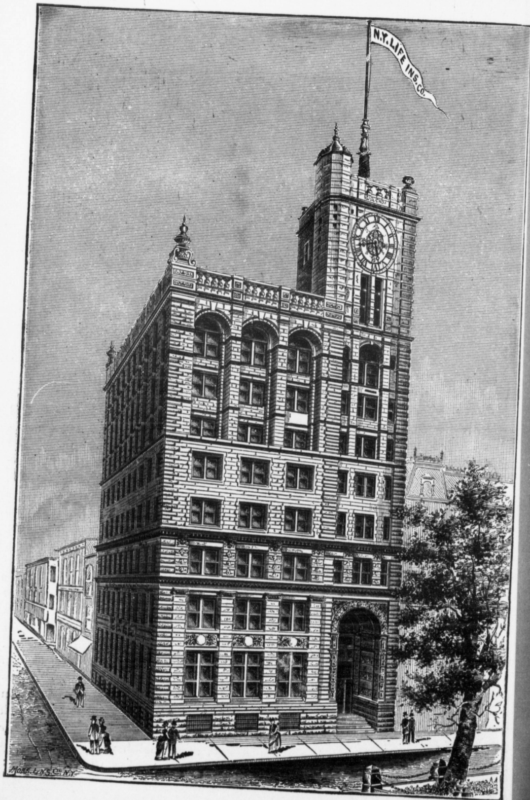
NEW YORK LIFE INSURANCE COMPANY'S BUILDING ERECTED 1888.
