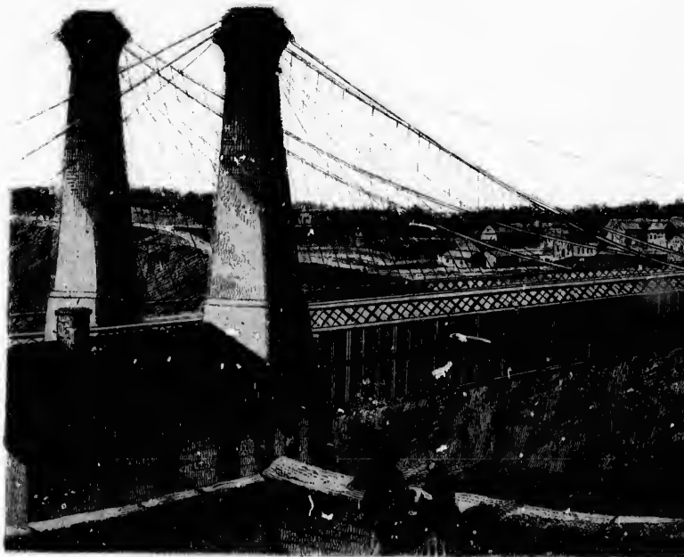
NIAGARA CAST IRON BRIDGE
