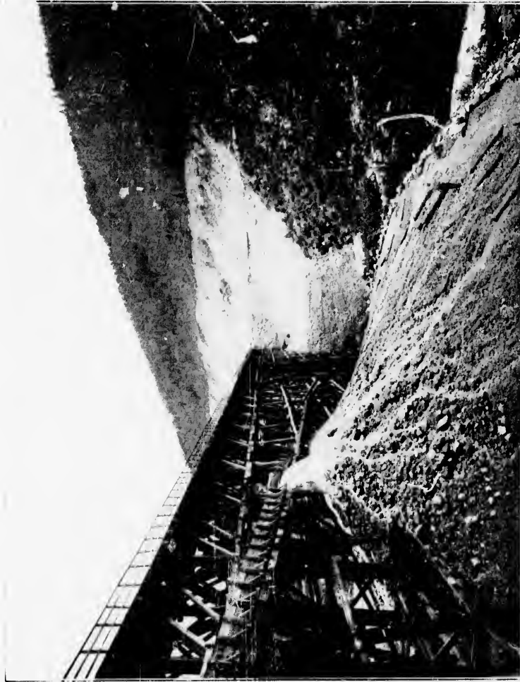
G. and W. S. FINE, JR. FIG. 10. GENERAL VIEW OF SLICE AND FILLING, MOUNTAIN CREEK, ROGERS' PASS
