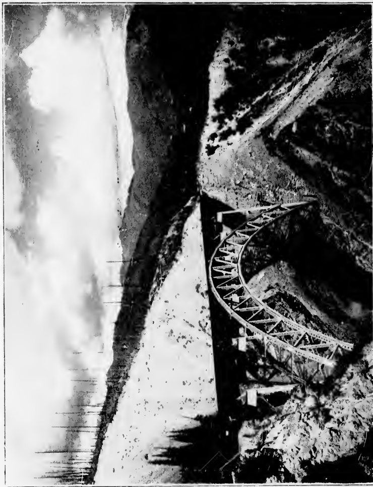
FIG. 7.—STONY CREEK BRIDGE, ROGERS' PASS. Height, 300 feet; span, 536 feet.
