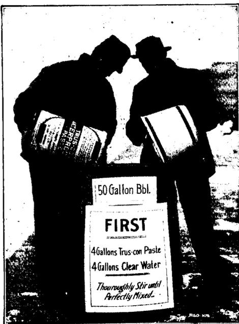
In the practical use of TRUS-CON WATERPROOFING PASTE best solution is obtained if one part of PASTE, either by weight or volume, is first thoroughly mixed with an EQUAL amount of clear water and then diluted as shown on next illustration.
