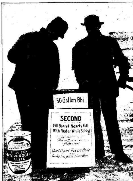
When equal parts of PASTE and water are evenly mixed add while stirring vigorously eleven additional parts of water, so as to give a final mixture of one (1) part of PASTE to twelve (12) parts of water.
