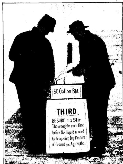
When mixture of PASTE and water is allowed to stand between batches it is advisable to stir before using to insure an even mixture throughout the entire work.
