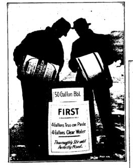
In the practical use of TRUS-CON WATERPROOFING PASTE best solution is obtained if one part of PASTE, either by weight or volume, is first thoroughly mixed with an EQUAL amount of clear water and then diluted as shown on next illustration.
