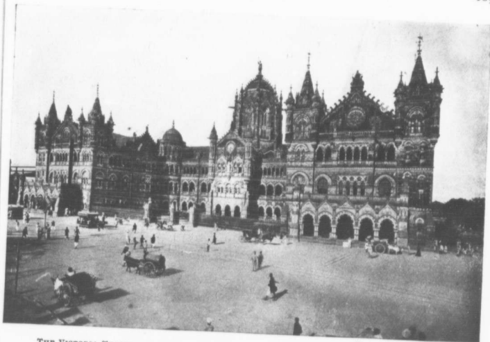
THE VICTORIA TERMINUS AND OFFICES OF THE GREAT INDIA PENINSULA RAILWAY, BOMBAY. This is probably the finest railway station in the world.
