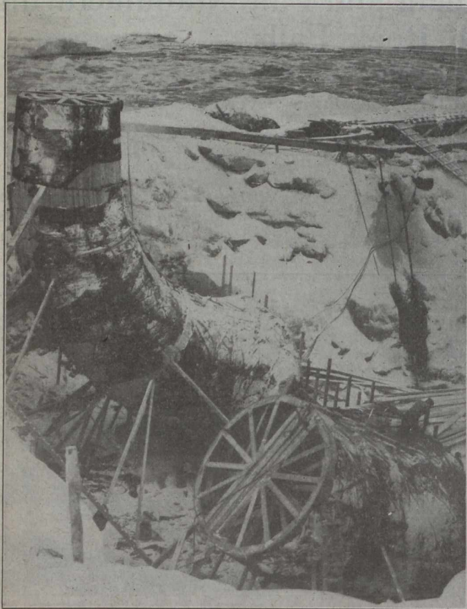
Installation of Draft Tube Forms
