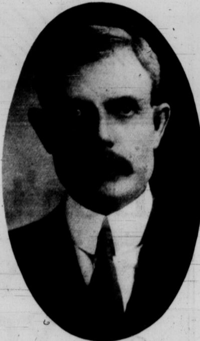
Mr. White, chief weighmaster at the terminal elevator
