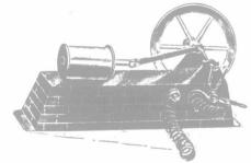
This is the Sayer Electric Engine, built on scientific lines and modeled after a modern Horizontal Corliss Steam Engine. The engine can be run in either direction and at different speeds by means of the controlling lever. It is the cheapest Electro Motor Engine It consumes but half ampere of current (about the same as a Miniature Battery Lamp). Two dry cells do the work.
