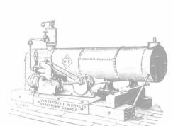
Portable Saw-Mill Engine.
