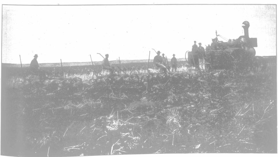
Plowing with Thirteen 14-inch Plows in Red River Gumbo Soil.
