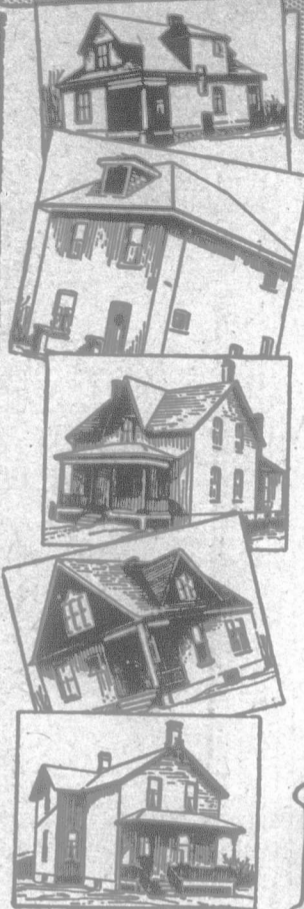
Five typical homes now heated by the "Hecla" Pipeless.
