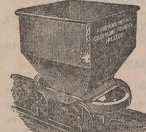
69—R. H.'s Improved Steel Hopper Wagon with Slide Door
