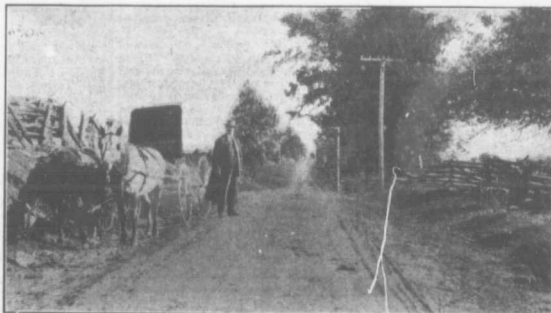
A GRAVELLED COUNTY ROAD IN HASTINGS
